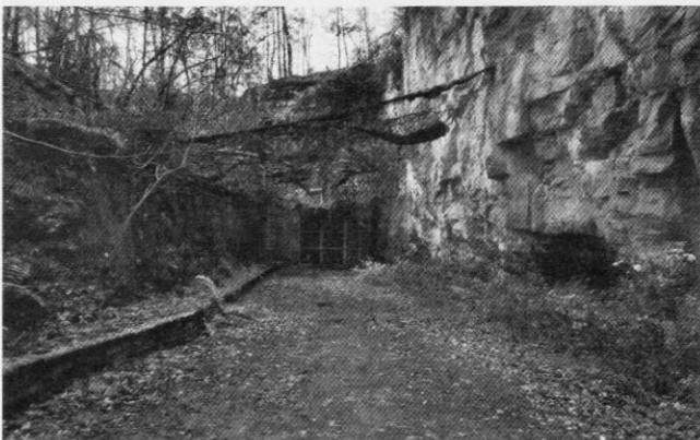
The personnel entrance (K on the plan). Photo Nick Catford
